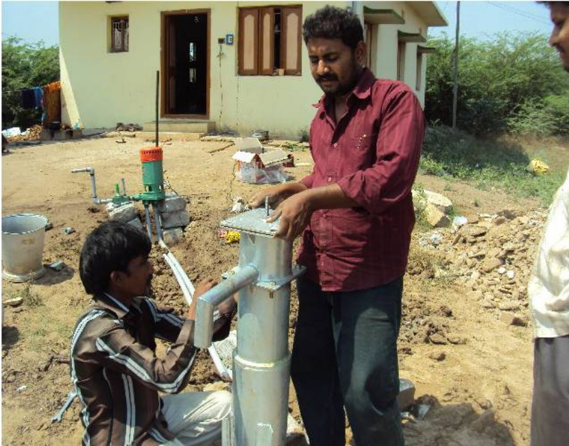
Project in Process; instillation of the new hand pump
