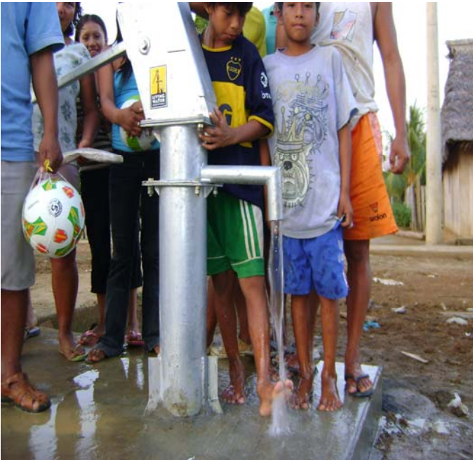
Community residents pumping clean drinking water
