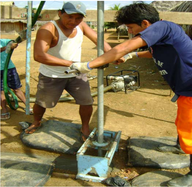
Project in Process
