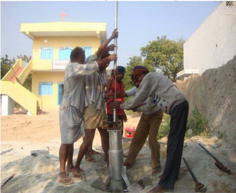
Project in Process
