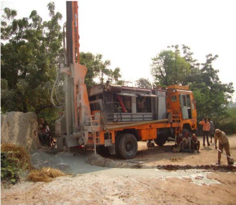
Project in Process
