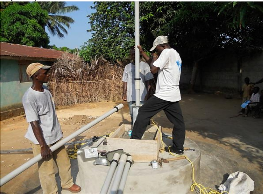
Project in process.
