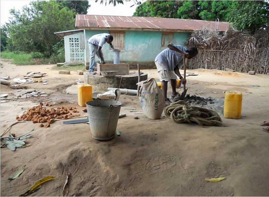
Project in process.
