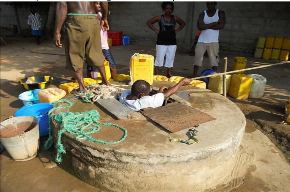
Project in process.
