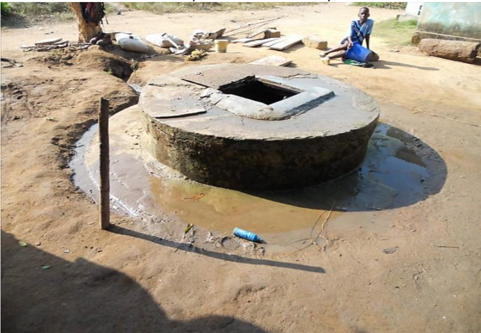
Previous water source, open and contaminated well.
