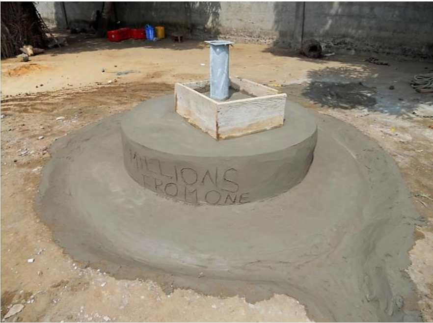
Project in process.
